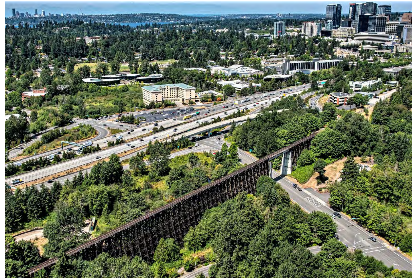
The Wilburton Trestle (Looking Northwest)
