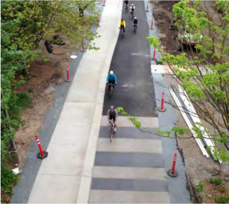
Transition Zone Treads at Intersections
